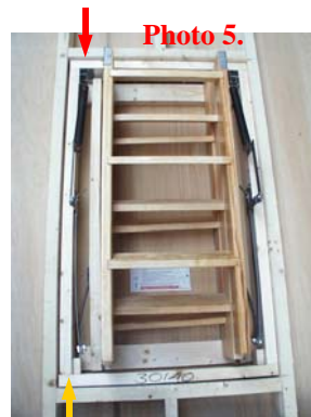
If frame is catching on the left, move frame forward at top left. (Red Arrow)
